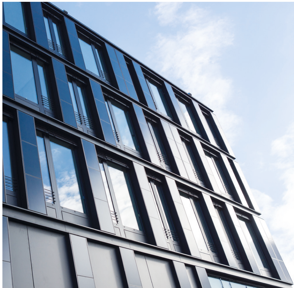
The ZSW institute's building in Stuttgart-Vaihingen features a striking CIGS facade. ▲
